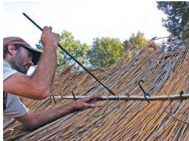
6 Thatchers Michael French and Lorin Johnson of Plimoth Plantation place bundled rolls at chimney base to hold next layer. Bundled rolls surround chimney perimeter.
