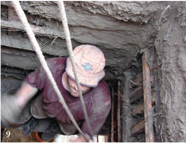
9 Jeremy R. Brown applies daub to framed, heavily lathed interior of spacious wood-framed chimney wetted down in Fig. 10, starting at top.
