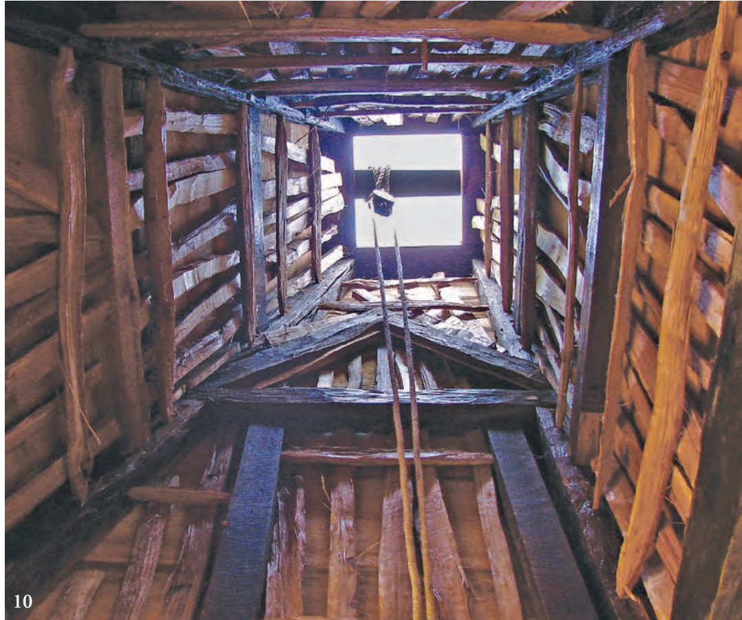
9 Jeremy R. Brown applies daub to framed, heavily lathed interior of spacious wood-framed chimney wetted down in Fig. 10, starting at top.
