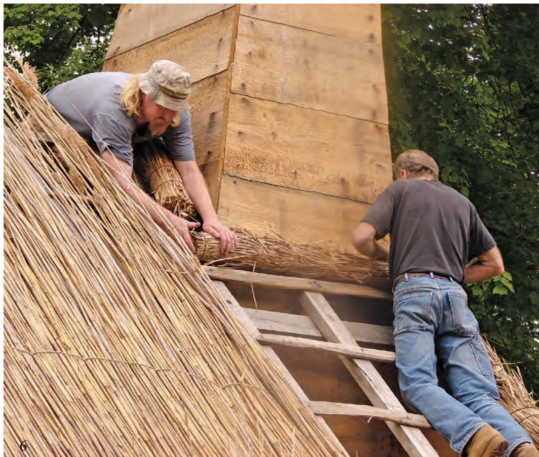
6 Thatchers Michael French and Lorin Johnson of Plimoth Plantation place bundled rolls at chimney base to hold next layer. Bundled rolls surround chimney perimeter.
